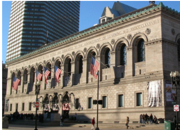
Boston Public Library McKim Building (1888, NR# 73000317) Boston, MA Restoration, Renovation and Alterations
